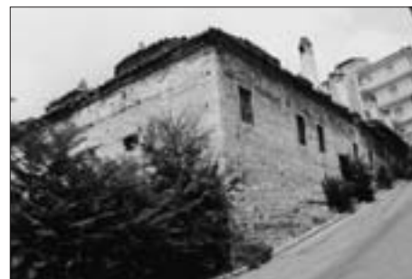
6. KASTORIA MEDRESE (UNDER RESTORATION)
